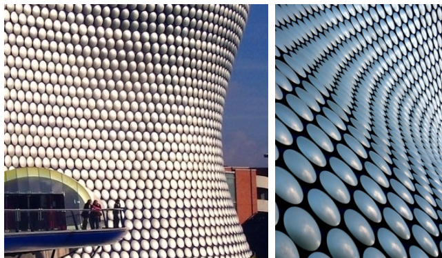
Figure 2: Arrangement of circles in freeform architecture. This image shows two different views of the Selfridges building, Birmingham, by Future Systems (right hand image courtesy P. Terjan).
