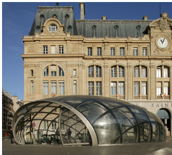
Figure 22: Repetition aids manufacturing efficiency. The lentille at Saint Lazare metro station is composed of a sphere and a torus, and has a rotational symmetry no longer apparent after panelization. This symmetry enabled the reuse of molds used in the manufacturing of glass panels (engineering and photo: RFR).
