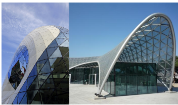
Figure 4: Optimization of triangle meshes: The Blob (left, photo by Evolute) in Eindhoven underwent Laplacian fairing subject to constraints like following floor slabs. Similar techniques were used for the Baku Funicular in 2012 (right, photo by T. Lorenz ZT).
