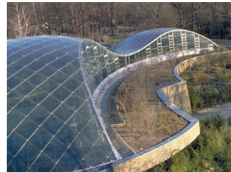
Figure 6: PQ meshes of simple geometry. Parallel translation of a polyline along another polyline generates a quad mesh with parallelogram faces (Hippo house, Berlin zoo, 1996. Photo and Engineering: Schlaich Bergermann & Partners).
