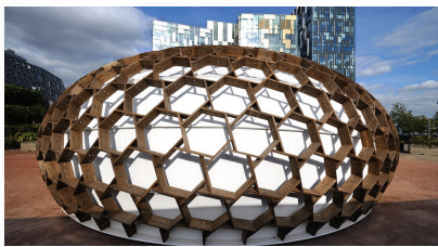
Figure 35: The hexagonal pattern exhibited by the KREOD pavilions is derived from the dual of a triangle mesh with the ball-packing property, leading to nice nodes and an even distribution of hexagons (image: KREOD).
