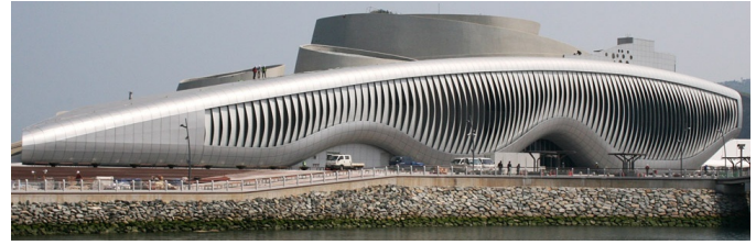
Figure 53: A kinetic facade based on bionic principles by Knippers Helbig, Stuttgart, is part of the 2012 One Ocean thematic pavilion by Soma Architecture, which has been built in Yeosu, South Korea.
