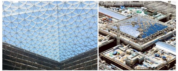
Figure 43: Yas Mall, Abu Dhabi: Gridshell with ornamental polyhedral pattern. Image at left: Stutzki Engineering Newsletter. Image at right, showing construction: Aldar.
