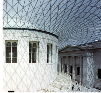
Figure 2: Triangle meshes in freeform architecture. Laying out a triangular pattern on a freeform surface and controlling its density and flow is a challenging problem successfully solved in 2000 by Chris Williams for the Great Court Roof of the British Museum in London (designed by Foster+Partners). Here dynamic relaxation was employed to aesthetically distribute the triangles (Photo: Waagner-Biro Stahlbau).
