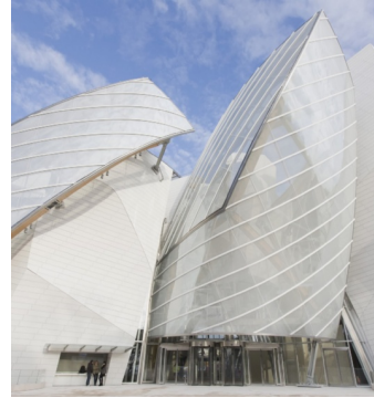
Figure 11: Each of the ‘sails’ of the Fondation Louis Vuitton by Frank Gehry consists of developable strips – for a mathematician this is an example of a semidiscrete conjugate surface. For the actual building, the strips were approximated by cylindrical glass panels (Photo: Mairie de Paris).
