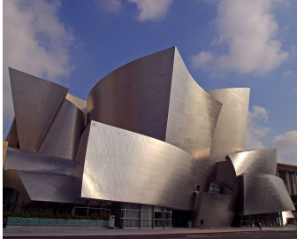
Figure 9: A pioneer of using developable freeform surfaces is Frank Gehry. A combination of physical and digital modeling has been used for the 1997 Guggenheim Museum in Bilbao as well as for other projects like the 2003 Walt Disney Concert Hall in Los Angeles (at left, photo by Jon Sullivan).
