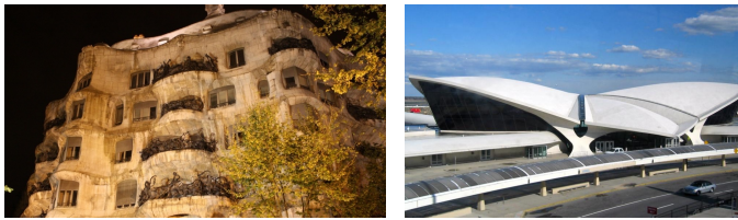
Figure 17: An early 20th century freeform geometry shaped in masonry is the 1910 Casa Milà in Barcelona by Antonio Gaudí (Photo at left by Kyle Taylor). Later, freeform shapes were realized at a grander scale in concrete, such as the TWA flight centre at JFK airport by Sarinen in 1962 (right).
