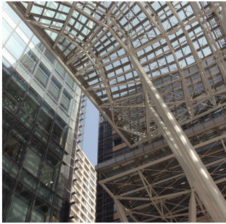
Figure 7: Example of a freeform PQ structure: The Roppongi Canopy at Tokyo Midtown Plaza, realized in 2005 by Buro Happold. Little documentation about this project is publicly available, but it appears to be based on a planar quad mesh following the principal curvature lines of the design surface.
