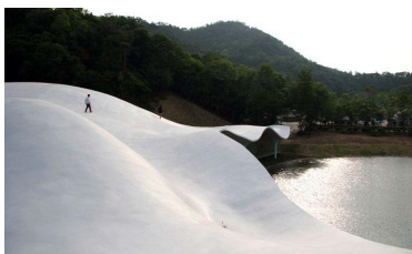
Figure 18: The 2006 Kakamigahara funeral hall by Toyo Ito is a freeform concrete shell without panels, still representing an instance of the “paneling problem” with respect to the formworks needed for pouring concrete (photo: Toyo Ito & Associates).
