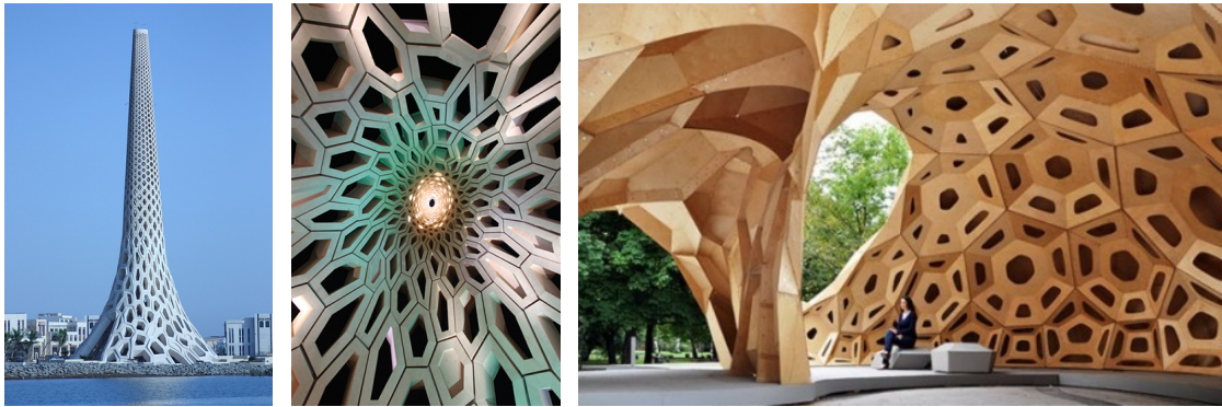
Figure 4: Hex-dominant structures. Left and center: The KAUST Breakwater Beacon at the entrance to the harbour of the King Abdullah University of Science and Technology in Saudi Arabia, by Urban Art Projects. Right: ICD/ITKE Research Pavilion 2011 at the University of Stuttgart.
