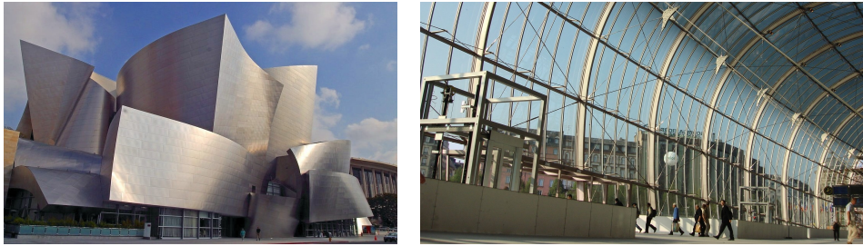
Figure 12. Single-curved surfaces . Left: The outer skin of the Disney concert hall in Los Angeles by Frank Gehry is covered by metal sheets and consists of approximately developable surfaces (image courtesy pdphoto.org ). Right: The glass canopy at the Strasbourg railway station exhibits “cold bent” glass panels (image courtesy RFR).
