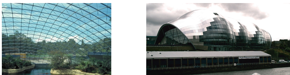
Figure 5. Not entirely freeform surfaces. Left: The hippo house in the Berlin zoo is based on a quadrilateral mesh with flat faces, but is not freeform in the strict sense. Its faces are parallelograms, so the mesh is generated by parallel translation of one polyline along another one. Mathematically, vertices v_{i,j} have the form v_{i,j} = a_i + b_j . Right: the Sage Gateshead building on the river Tyne, UK, is based on a sequence of polylines which are scaled images of each other, similar to a mesh with rotational symmetry.
