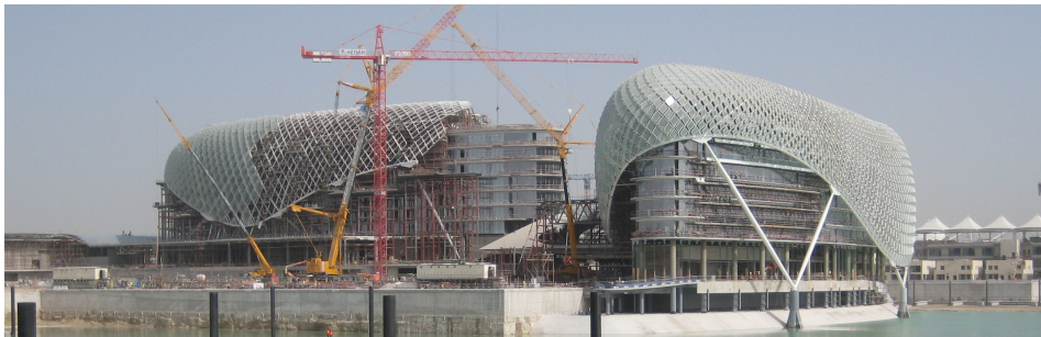
Figure 1. Freeform architecture. The Yas Marina Hotel in Abu Dhabi illustrates the decomposition of a smooth skin into straight elements which are arranged in the manner of a torsion-free support structure. The practical implication of this geometric term is easy manufacturing of nodes (image courtesy Waagner-Biro Stahlbau).
