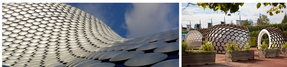
Figure 16. Regular Patterns. Left : The facade of Selfridges, Birmingham (UK) is decorated with a circle pattern. Right : The “Kreod” pavilions, London, are derived from the support structure defined by a triangle mesh with incircle packing property.
