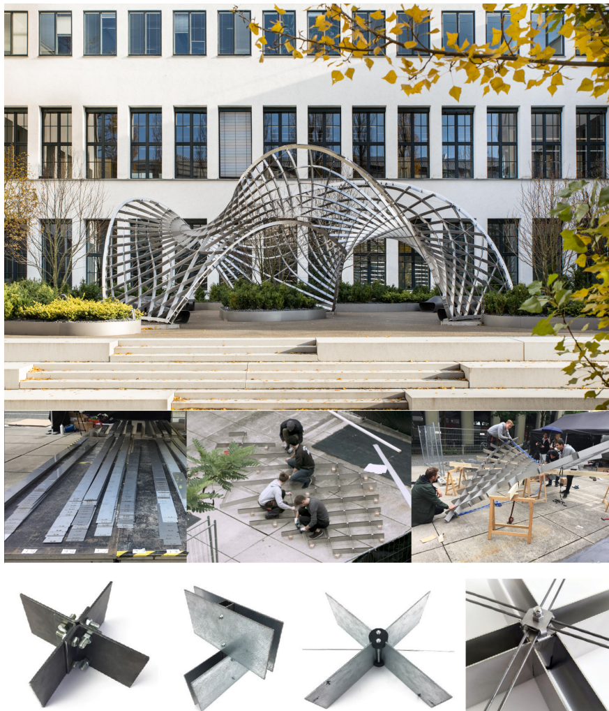
Fig. 1: An asymptotic gridshell (top) [1]. Straight lamellas (middle) follow asymptotic curves of the reference surface and intersect under a right angle. This simplifies the manufacturing process as all steel joints (bottom) are identical but forces the reference surface to be a Euclidean minimal surface. If the intersection angle is constant and not right, then the joints are still identical, and we get more general surfaces: ones with a constant ratio of principal curvatures.
