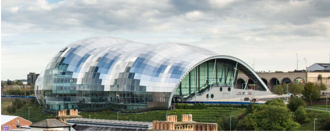
Fig. 2. Quadrilateral meshes with planar polylines. The Sage Gateshead concert venue, completed in 2004 and designed by Foster+Partners, is based on a quad mesh with planar faces and planar mesh parameter lines.
