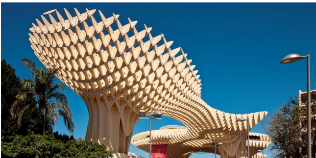
Fig. 3. The Metropol Parasol in Seville, Spain, designed by Jürgen Mayer and completed 2011 not features planar mesh parameter lines. The planes carrying parameter are structural elements.
