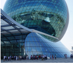
Fig. 2. Spherical glass panels are used by the Nur Alem Museum of Future Energy in Astana, Kazakhstan.
